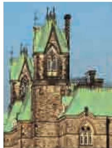
Figure 6.7 Although this green roof may contain some copper(II) oxide, it is mostly composed of basic copper sulfates and carbonates that form when the copper reacts with acid precipitation.
