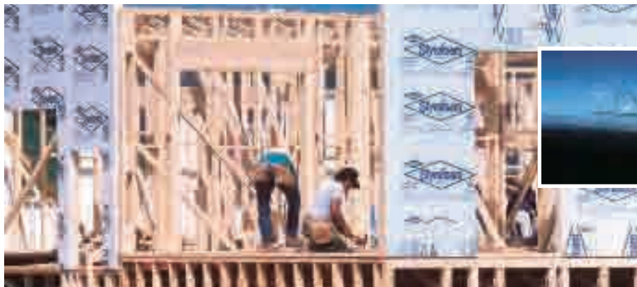
Figure 14.27 Polystyrene foam insulation, such as Styrofoam™, prevents heat flow and does not absorb water.
